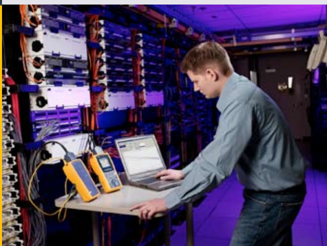
DTX-1800 com Kit DTX 10 Gigabit para testar performance Alien Crosstalk
